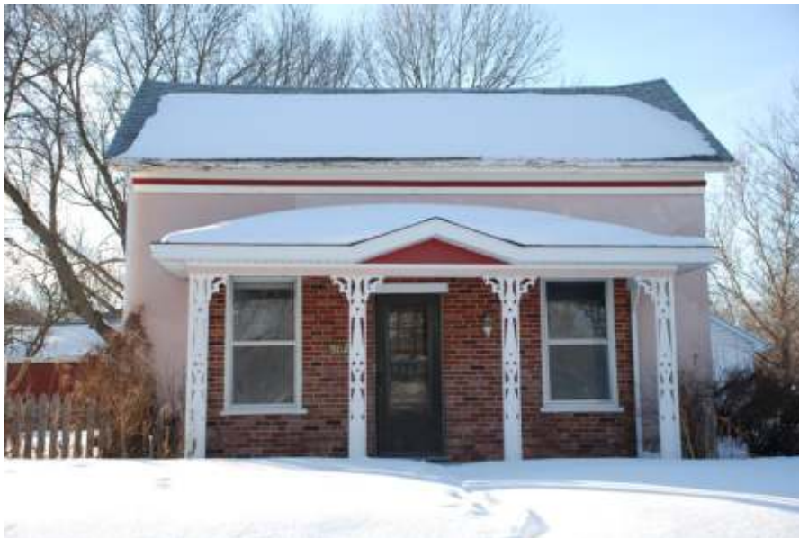
House, 502 1st St SW (1880), determined individually NRHP-eligible by SHPO, Criterion A
