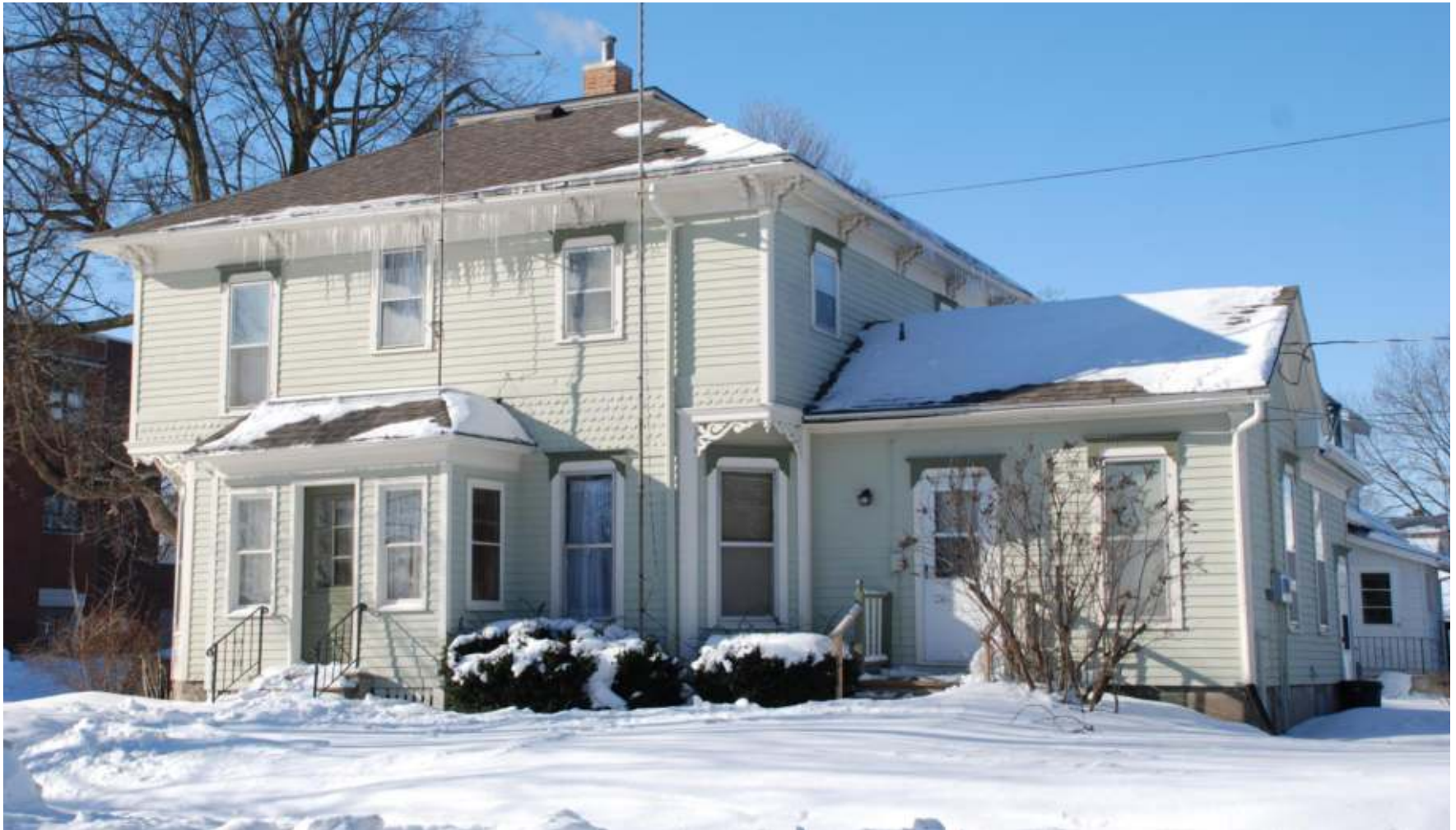
House, 303 3rd St NW (1897), Northwest Historic District, Waverly, potentially individually NRHP-eligible and contributing
