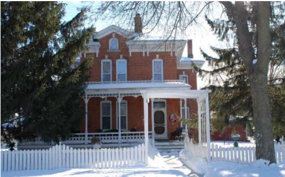
House, 401 2nd Ave SW (1876), potentially individually NRHP-eligible
