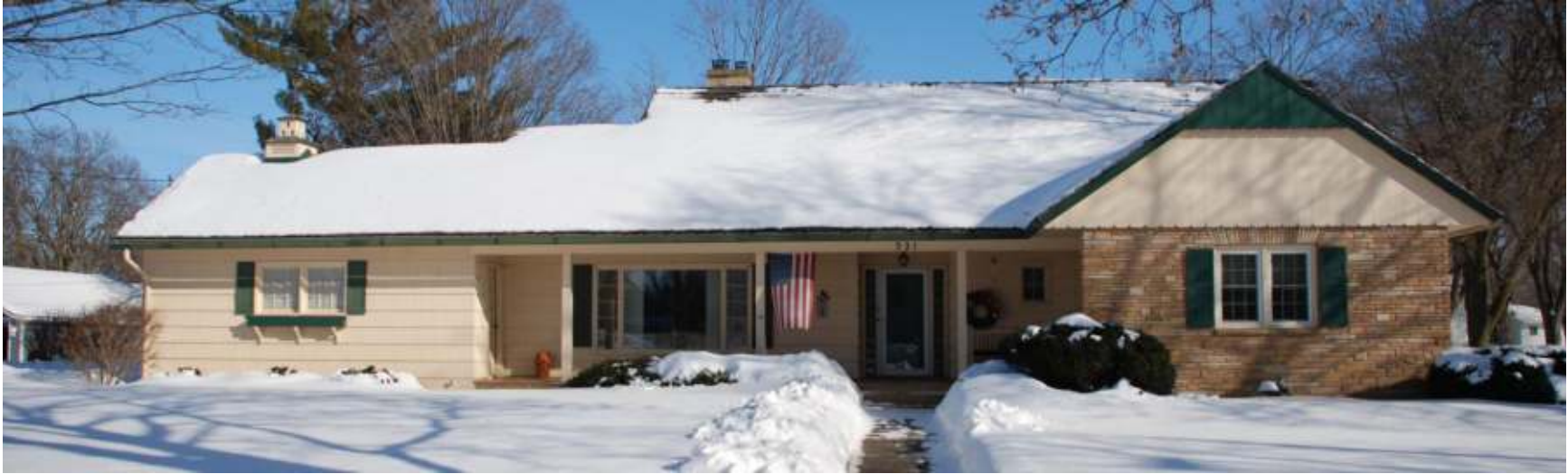
House, 321 8th St SW (1948), potentially individually NRHP-eligible
