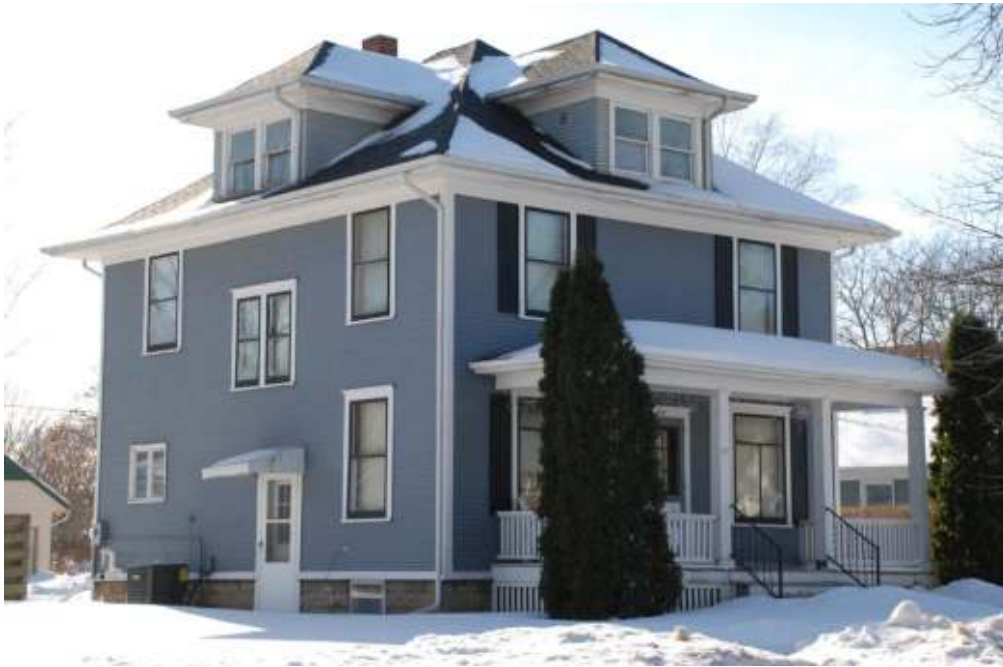
House, 717 2nd Ave SW (1913), potentially individually NRHP-eligible
