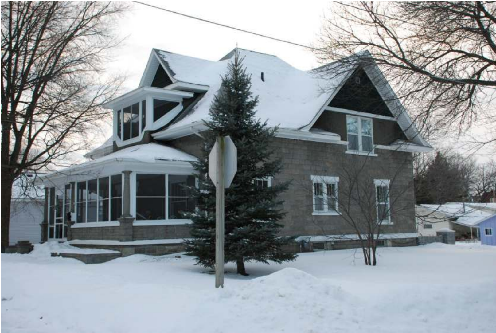
House, 323 5th St NW (1910), Northwest Historic District, Waverly, potentially individually NRHP-eligible and contributing
