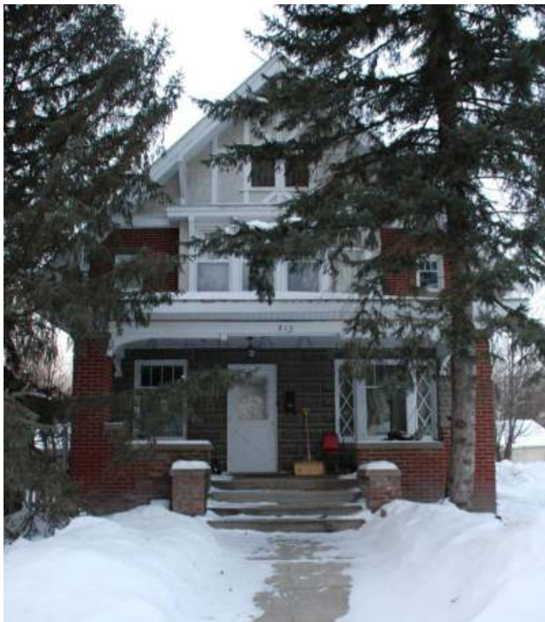
House, 213 5th St NW (1910), Northwest Historic District, Waverly, potentially individually NRHP-eligible and contributing
