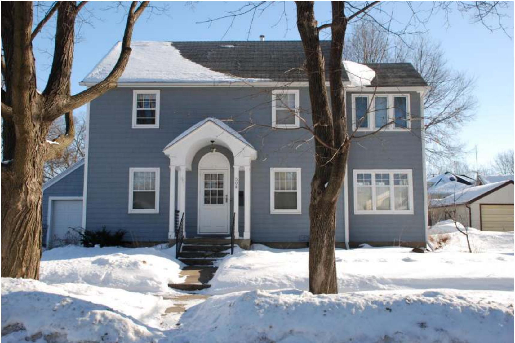
House, 508 4th St NW (1935), Northwest Historic District, Waverly, potentially individually NRHP-eligible and contributing
