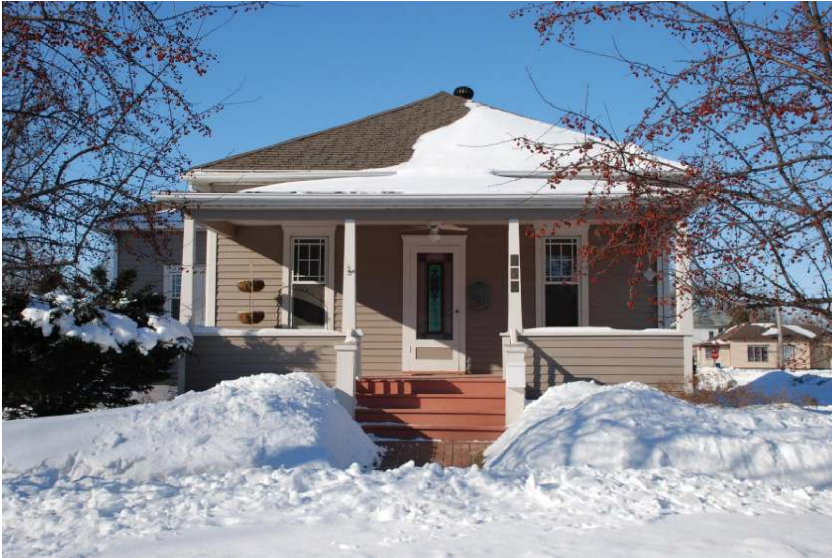
House, 523 4th St NW (1908), Northwest Historic District, Waverly, potentially individually NRHP-eligible and contributing
