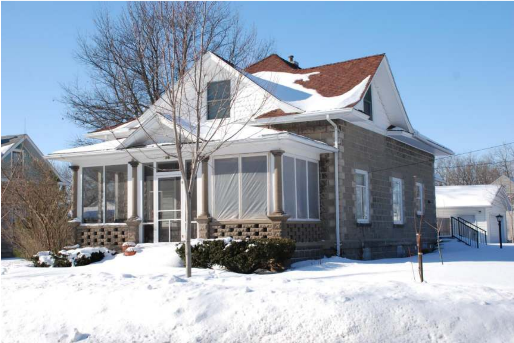
House, 623 3rd St NW (1905), Northwest Historic District, Waverly, potentially individually NRHP-eligible and contributing
