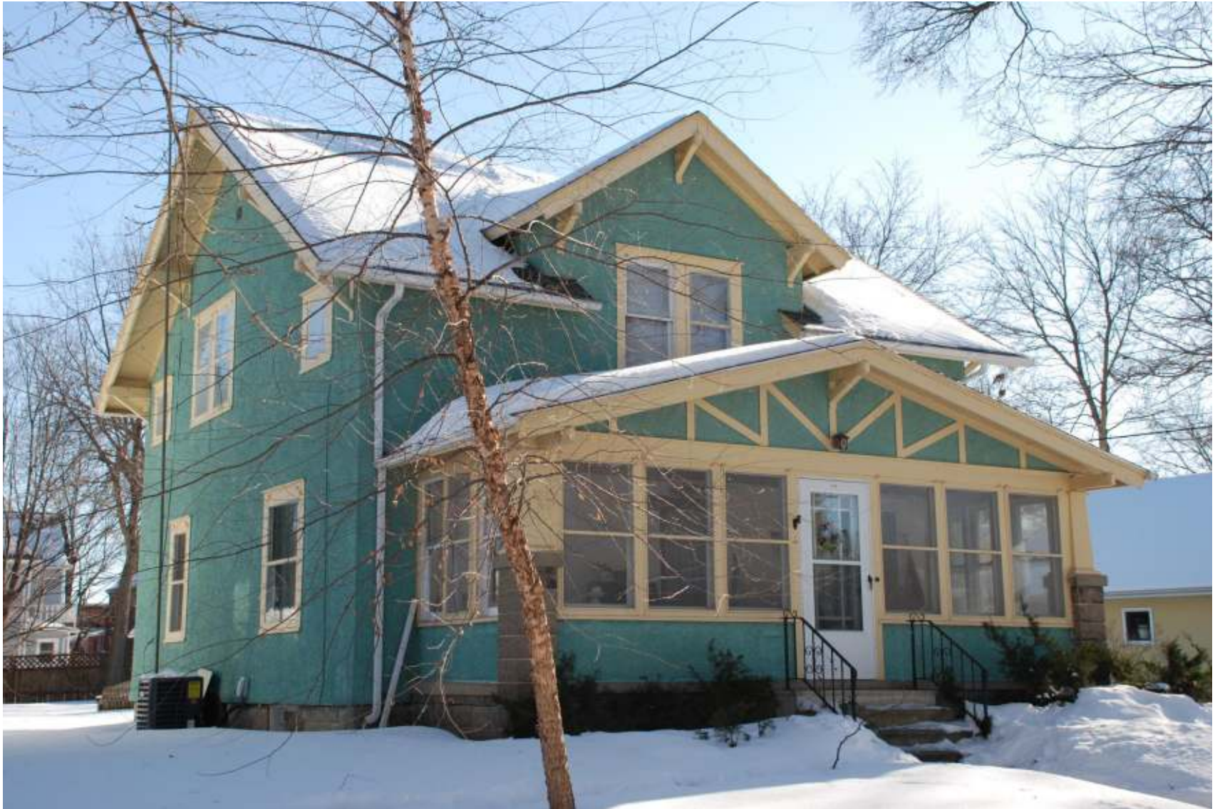
House, 316 3rd St NW (1920), Northwest Historic District, Waverly, potentially individually NRHP-eligible and contributing
