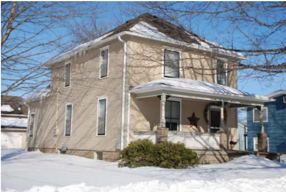
House, 420 5th Ave SW (1910), potentially individually NRHP-eligible
