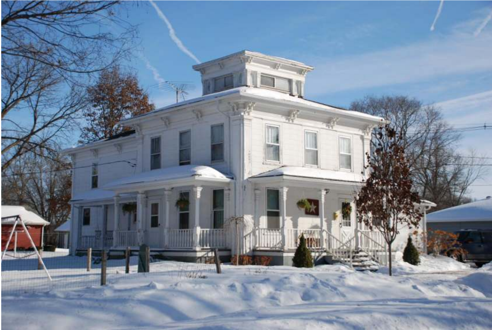
House, 507 2nd St SW (1880), potentially individually NRHP-eligible
