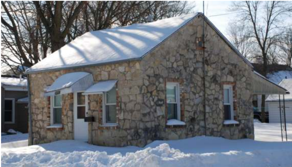
House, 214 7th St SW (1941), potentially individually NRHP-eligible
