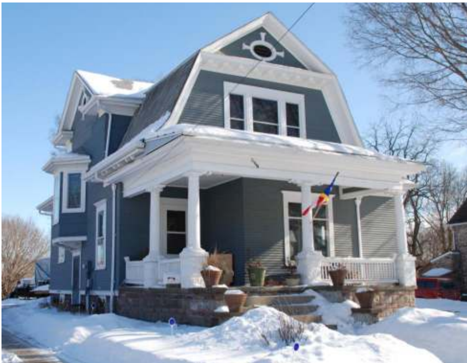
House, 407 3rd St SE (1910), Southeast/Old Fourth Ward Historic District, Waverly, potentially individually NRHP-eligible and contributing
