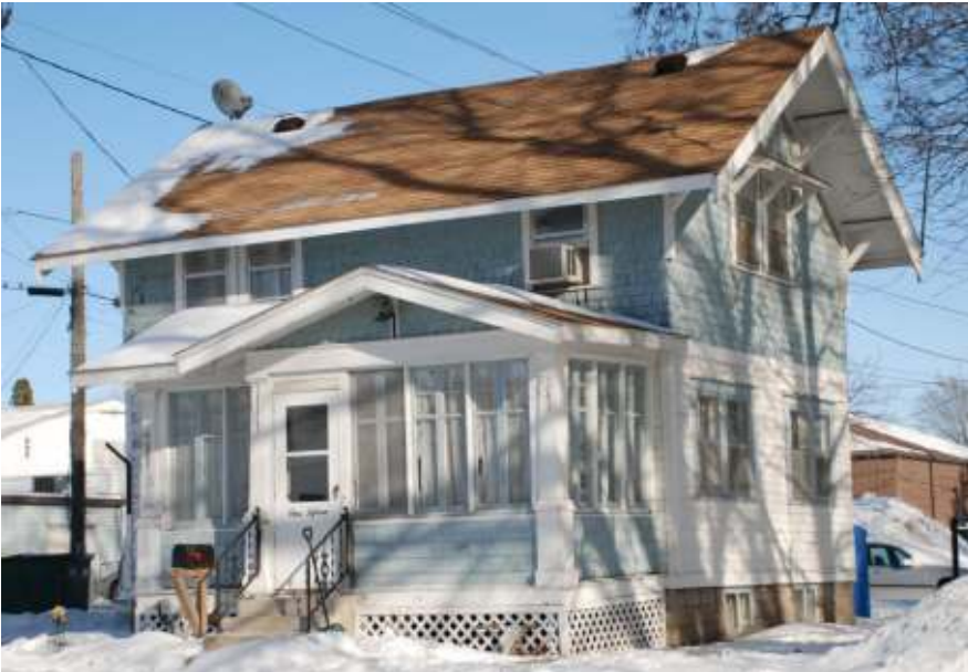
House, 115 3rd St SW (1865), potentially individually NRHP-eligible
