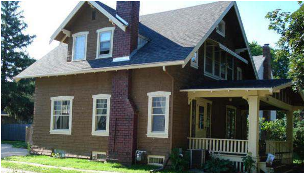
House, 215 3rd St SW (1916), potentially individually NRHP-eligible (RSDE Photograph)
