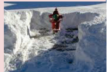
In the event of a fire, this hydrant is ready for use by the Waverly Municipal Fire Department.
