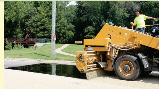
Contractor placing rock over oiled street. As soon as the rock has been placed on street, vehicles may drive slowly on the new surface.
