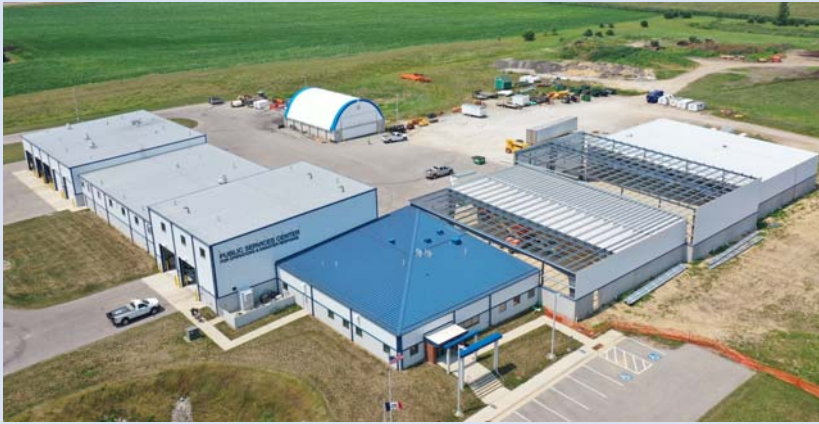
Construction progress at the Public Services Center.
