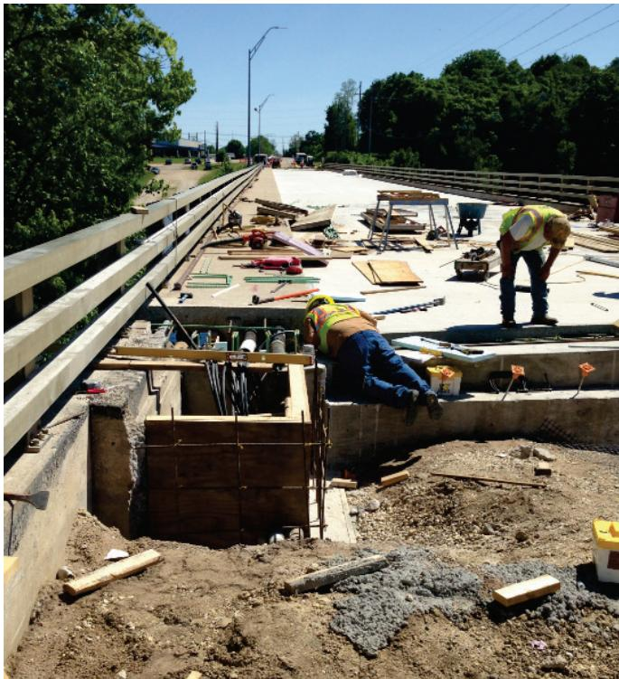
*The north side utility vault is being rebuilt so the lid is flush with the sidewalk.*
