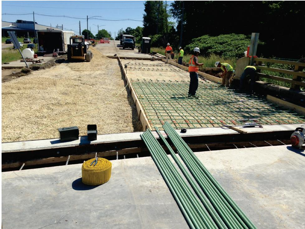
*Workers place and tie reinforcing bars for the roadway approach on the south end of the bridge.*
