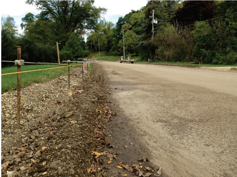
*String line is used to guide the paving machine and maintain the proper thickness of concrete.*
