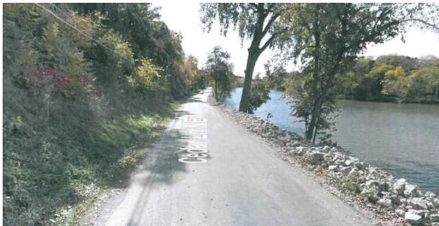
Two different roadway cross sections will be utilized. As shown above, the flat wide section of Cedar Lane will have 10-foot wide driving lanes and 5-foot wide paved shoulders. As shown left, the rolling narrow section of Cedar Lane will have 10-foot wide driving lanes and 2-foot wide curb & gutters. Given the limited available space, cars, bikes and pedestrians must continue to share the road.
