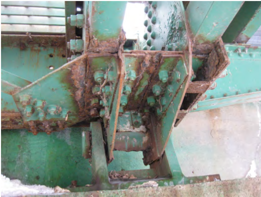
Figure 1 - Example Deterioration around Bearing
