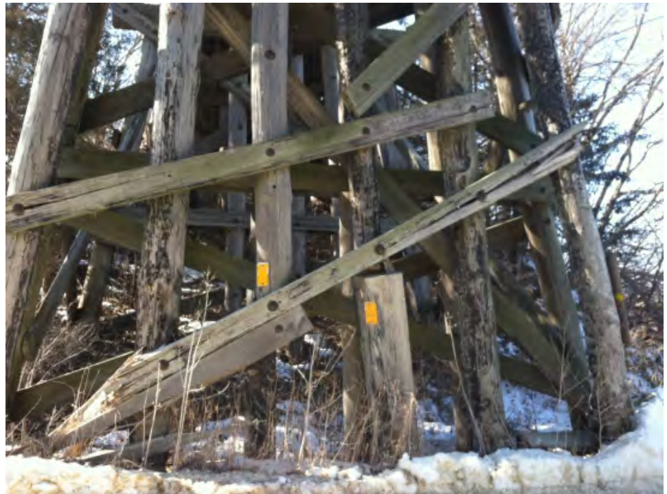
Photo No. 1 – Ivanhoe Pier 3
