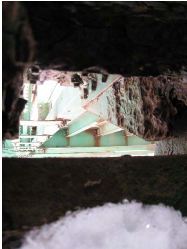
Figure 9 - Example Deterioration Above Bearing
