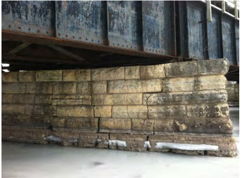
Photo No. 3 – Cedar River Pier
