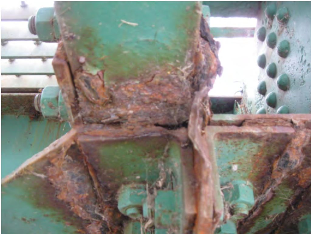
Figure 13 - Example Deterioration at Bottom Chord
