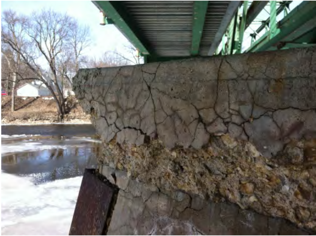
Figure 23 – Deterioration at South Pier (2013 Photo)
