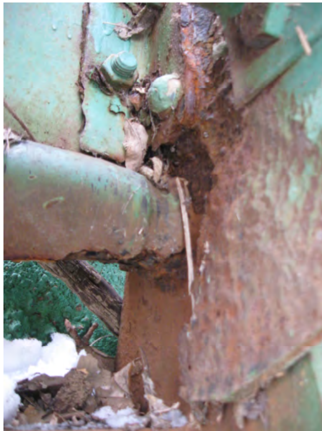
Figure 2 - Example Deterioration at Bearing
