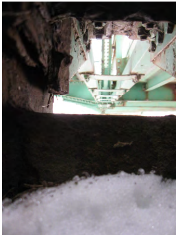
Figure 8 - Example Deterioration Above Bearing
