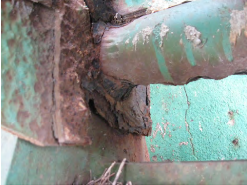
Figure 3 - Example Deterioration at Bearing
