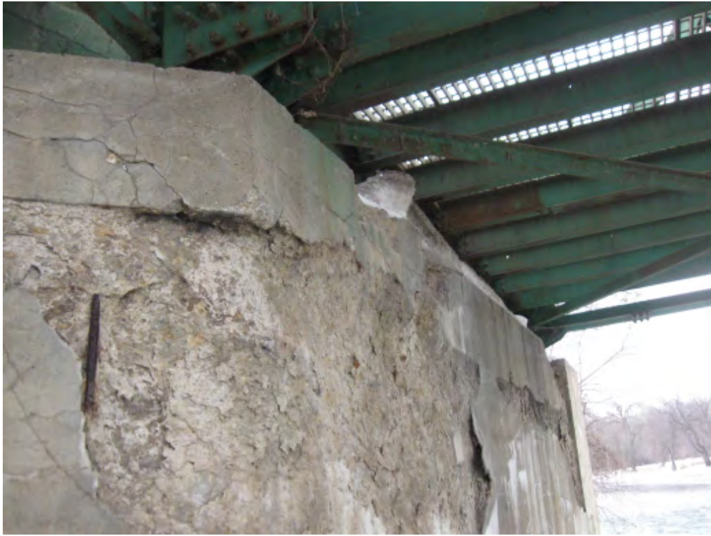
Figure 19 – Deterioration at North Abutment
