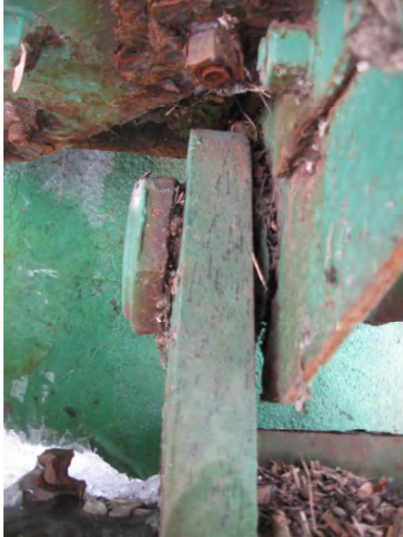
Figure 5 - Example Deterioration at Bearing
