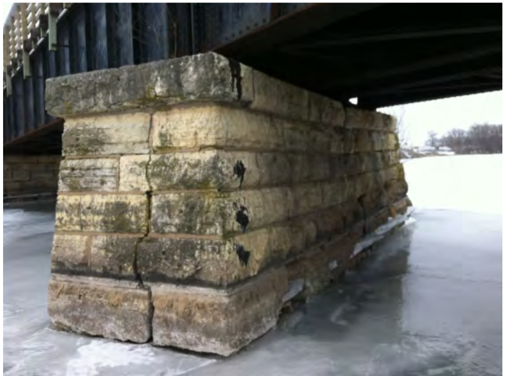
Photo No. 4 – Cedar River Pier
