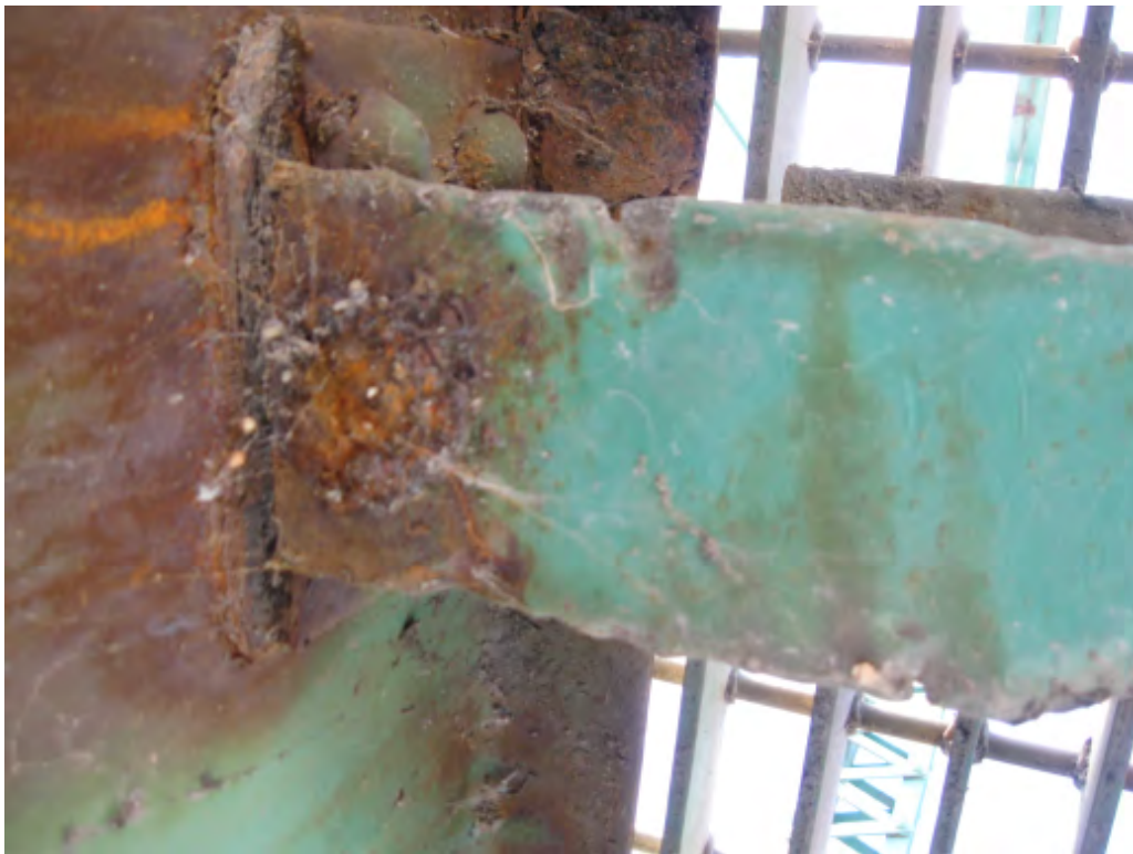
Figure 18 - Example Deterioration at Stringer Connection
