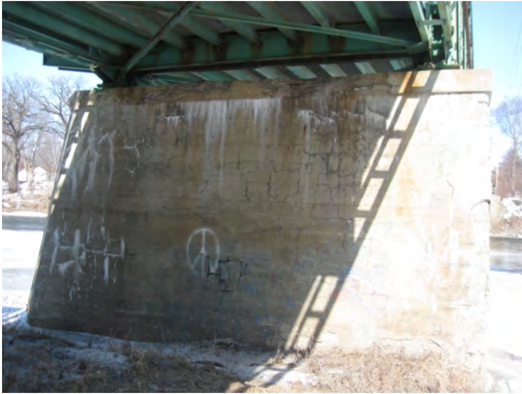
Figure 21 – Deterioration at South Pier
