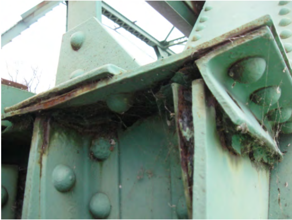
Figure 11 - Example Deterioration Above Bearing
