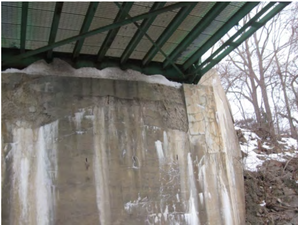
Figure 20 – Deterioration at North Abutment
