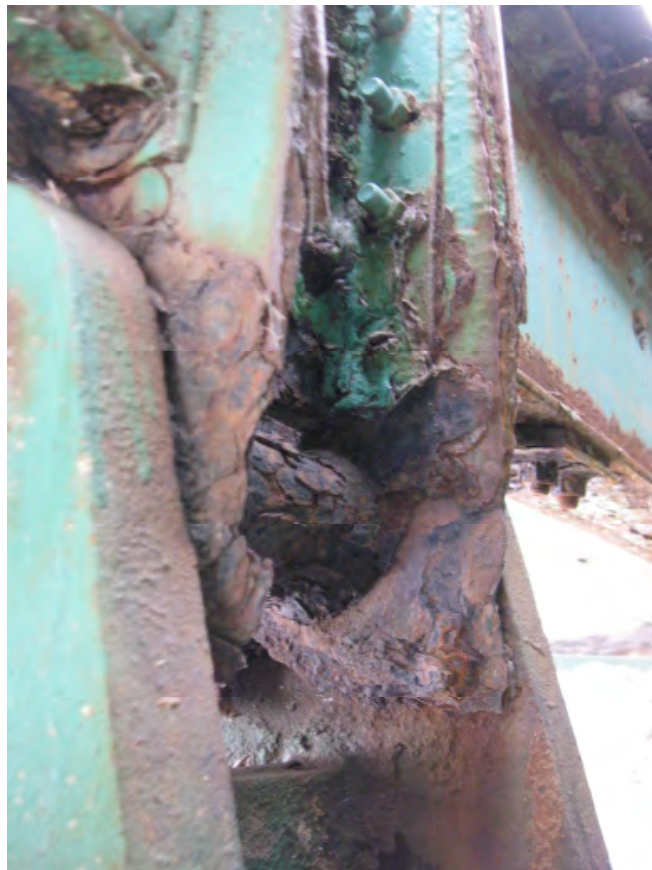
Figure 4 - Example Deterioration at Bearing
