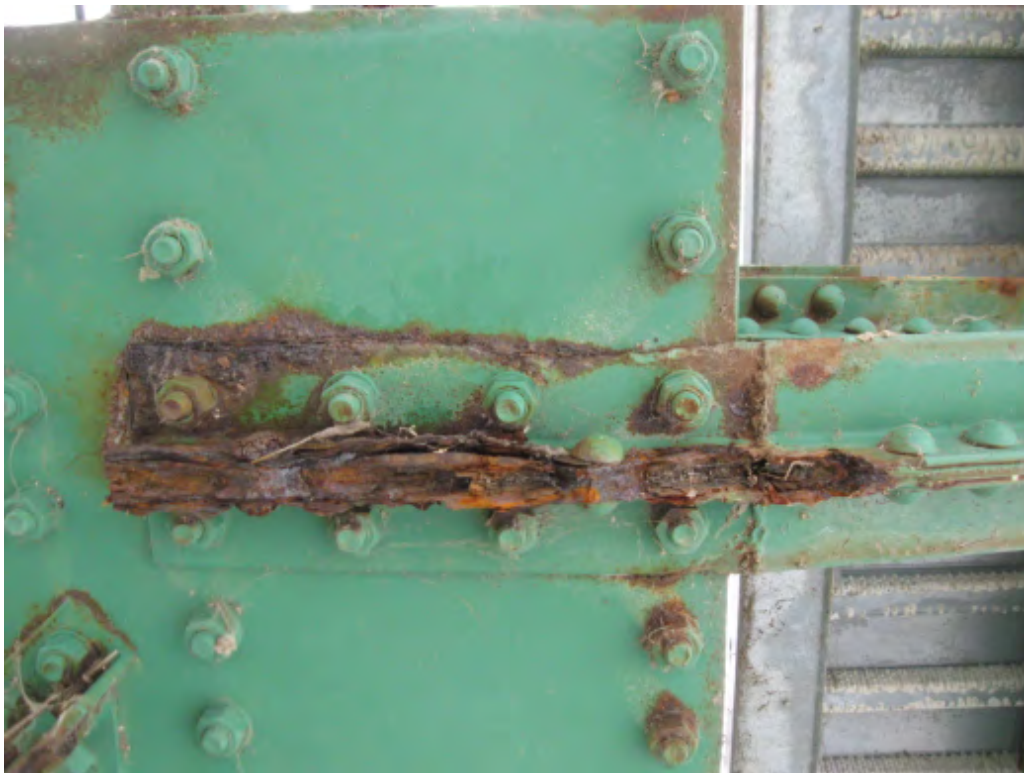
Figure 14 - Example Deterioration at Lower Sidewalk Connection
