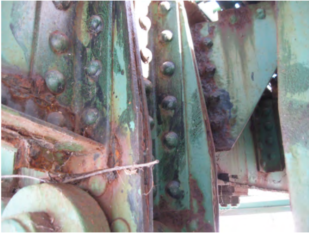
Figure 7 - Example Deterioration Above Bearing
