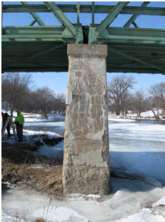
Figure 22 – Deterioration at South Pier
