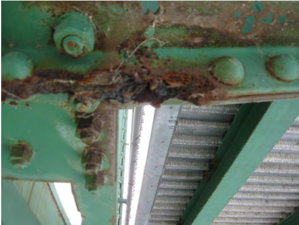
Figure 15 - Example Deterioration at Lower Sidewalk Connection
