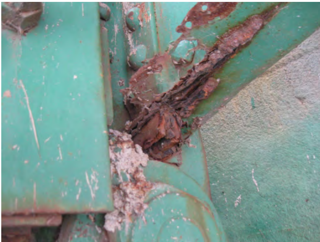
Figure 10 - Example Deterioration Above Bearing
