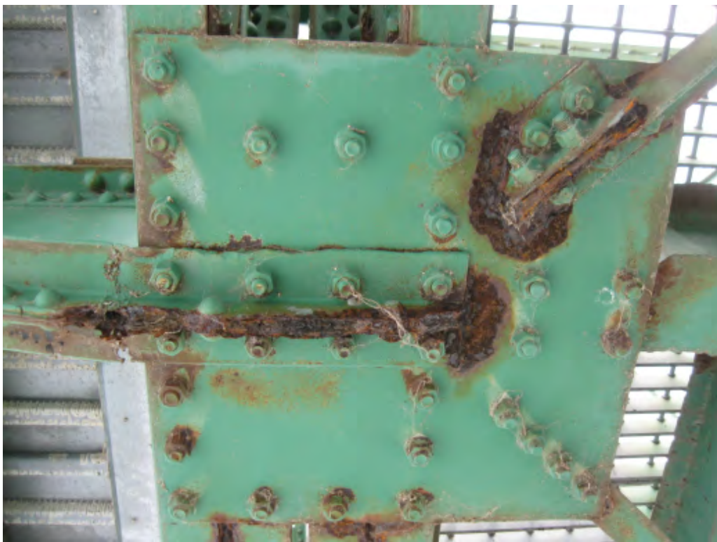
Figure 16 - Example Deterioration at Lower Horizontal Gusset Plate
