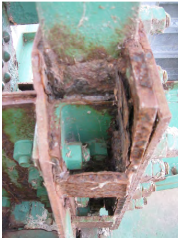
Figure 12 - Example Deterioration at Bottom Chord
