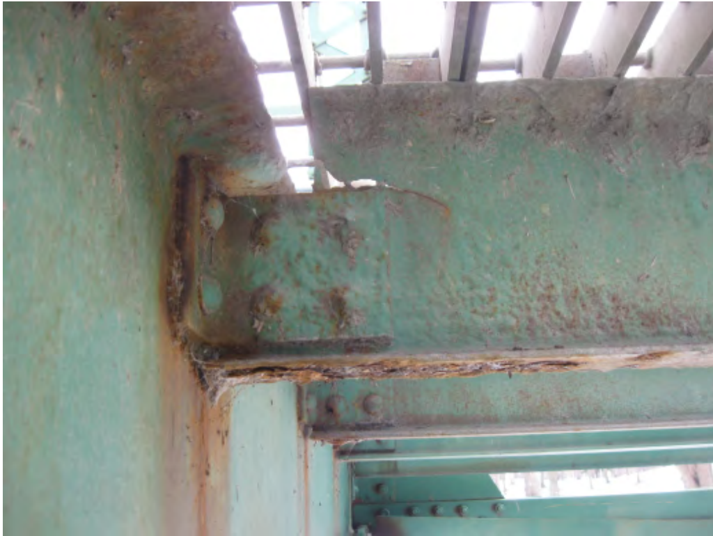
Figure 17 - Crack Progression in Stringer Web
