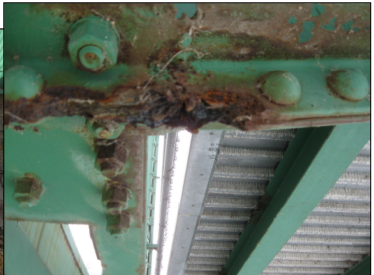
Deterioration at Lower Sidewalk Connection
