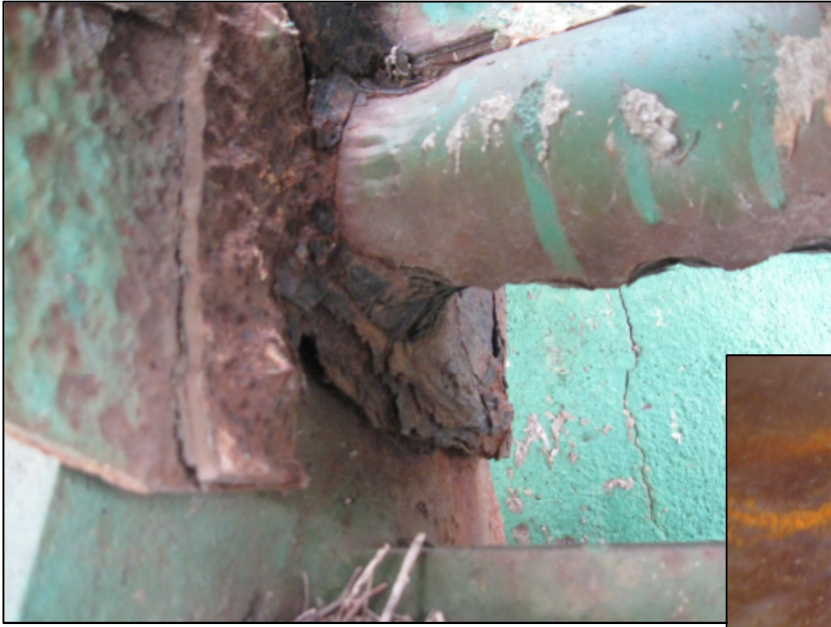
Deterioration at Bearing Which Supports the Bridge Span
