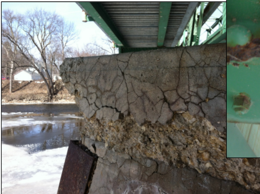
Deterioration of the South Pier Cap that Supports Two Bridge Spans
