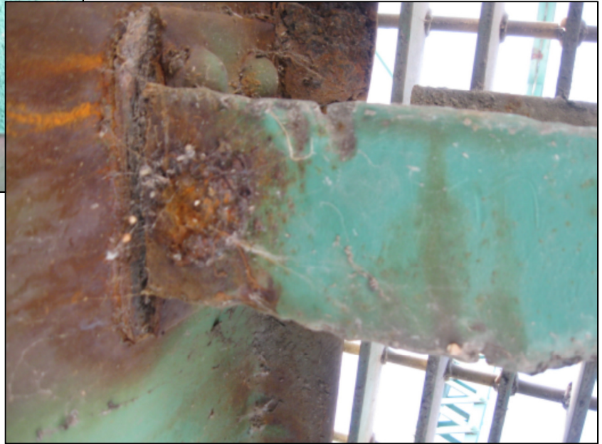
Deterioration at Stringer Connection Supporting the Metal Deck
