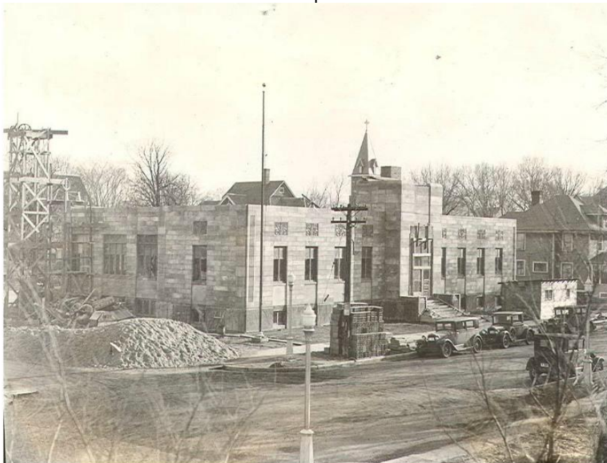
Historic photograph of the building under construction, 1932, taken from http://communitywebshots.com on 2/8/2012.
