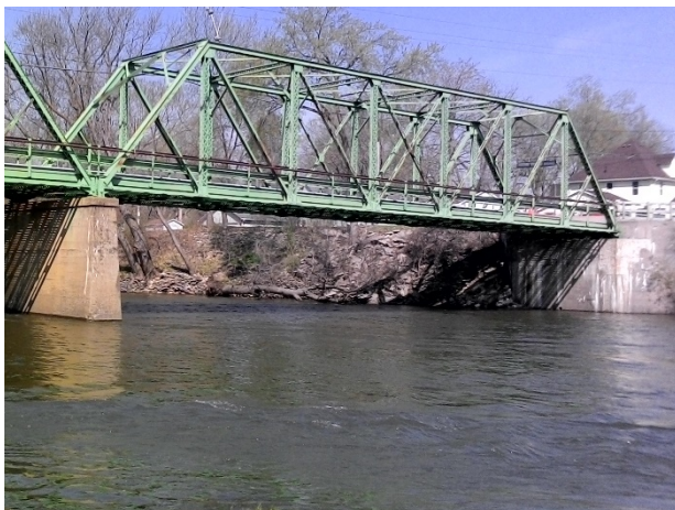
East Elevation – North Span
