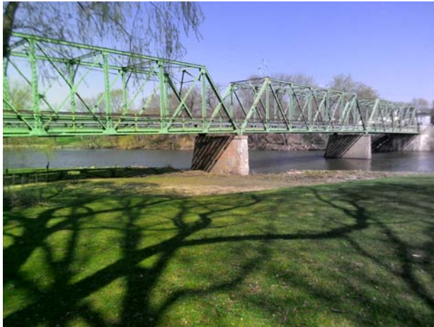
East Elevation from South Embankment
