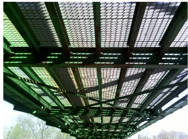
South Span Floor System Looking North
