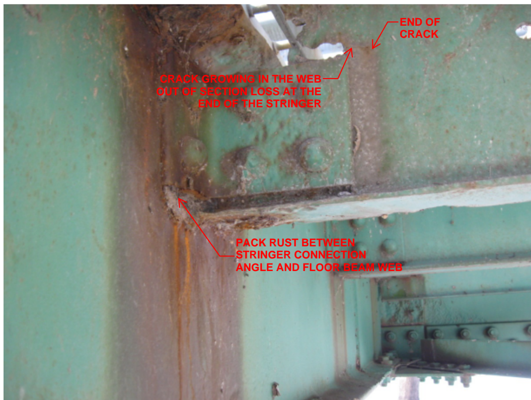
Figure 2: Crack at Stringer End
