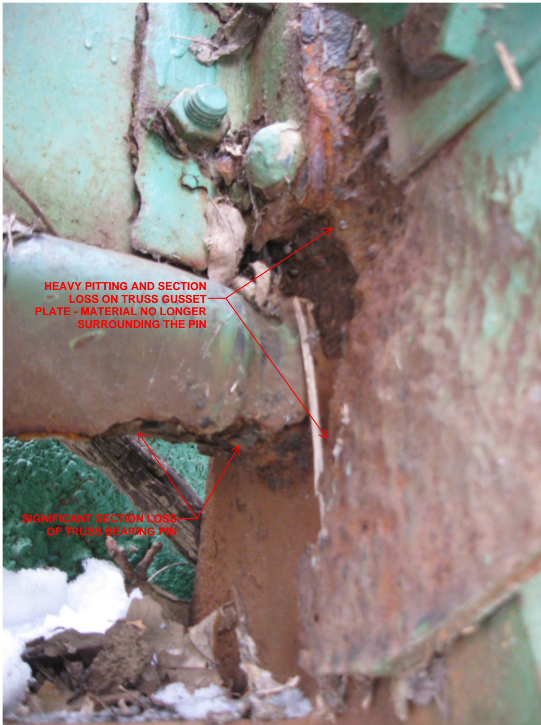
Figure 3: Deterioation at Bearing - Truss Gusset Plate Not Connected to Pin
