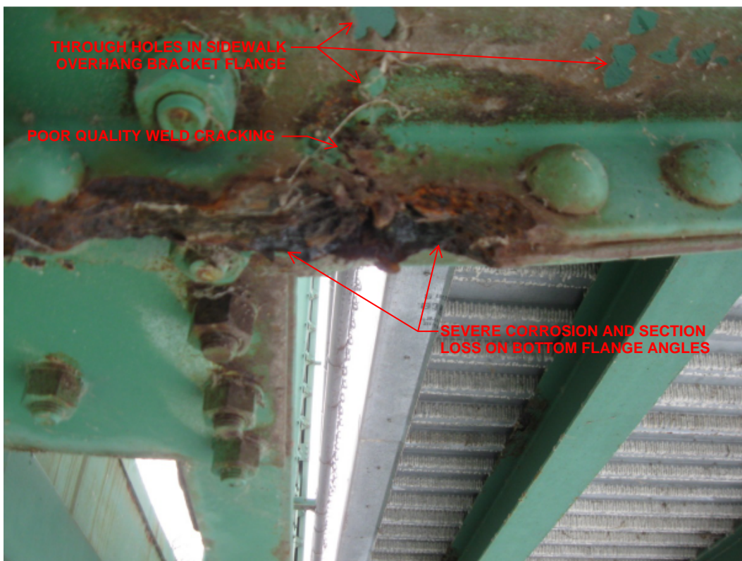
Figure 5: Bottom View of Sidewalk Overhang Bracket
