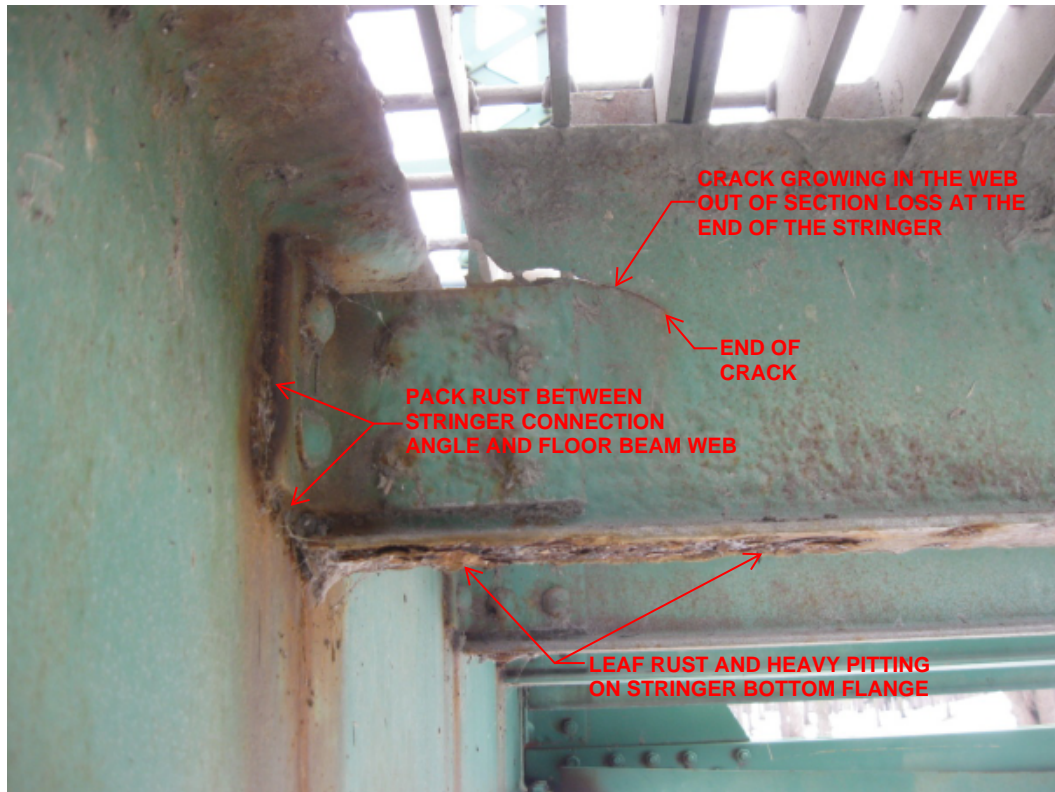
Figure 1: Crack at Stringer End
