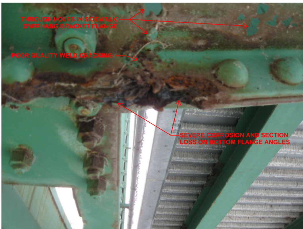
Figure 5: Bottom View of Sidewalk Overhang Bracket
