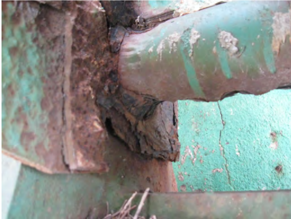
Figure 3 - Example Deterioration at Bearing
