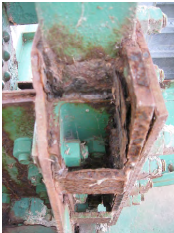
Figure 12 - Example Deterioration at Bottom Chord
