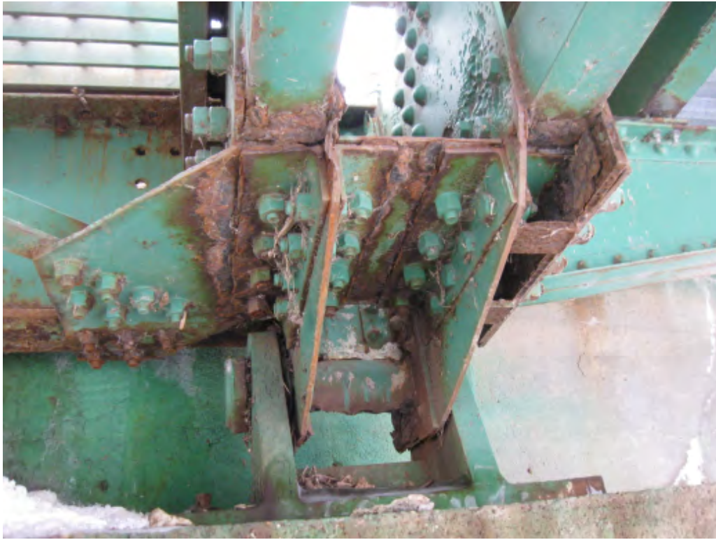
Figure 1 - Example Deterioration around Bearing
