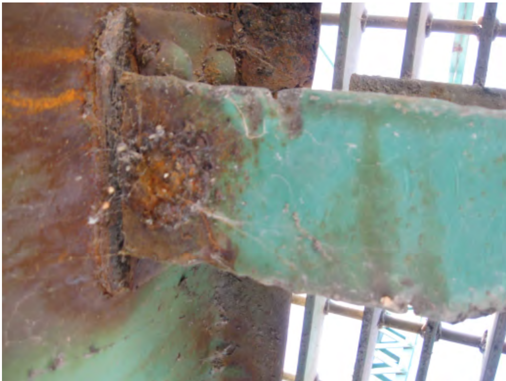
Figure 18 – Example Deterioration at Stringer Connection
