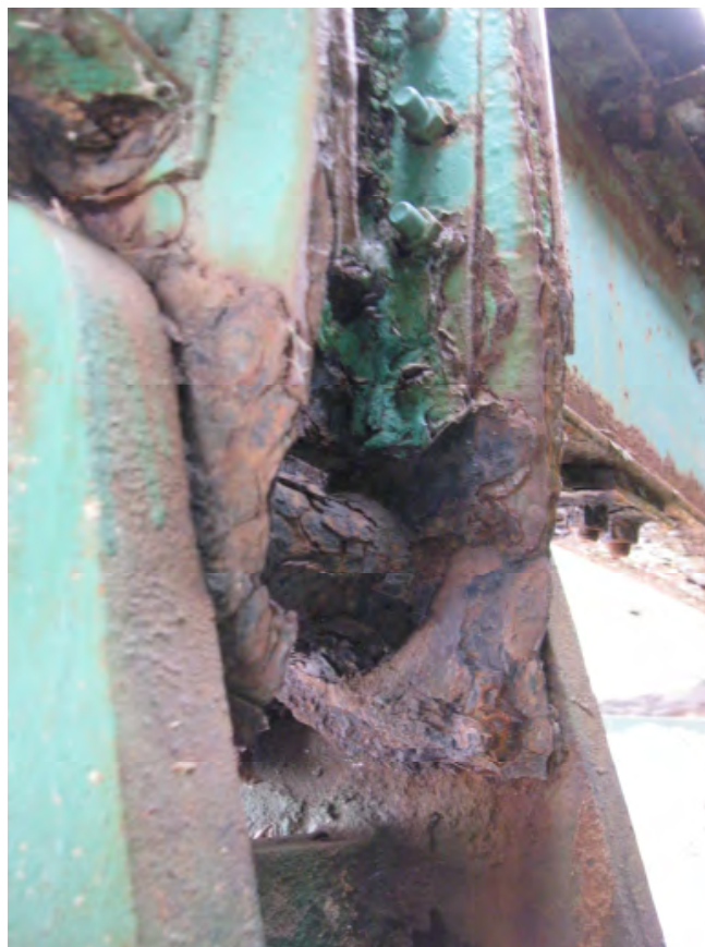
Figure 4 - Example Deterioration at Bearing
