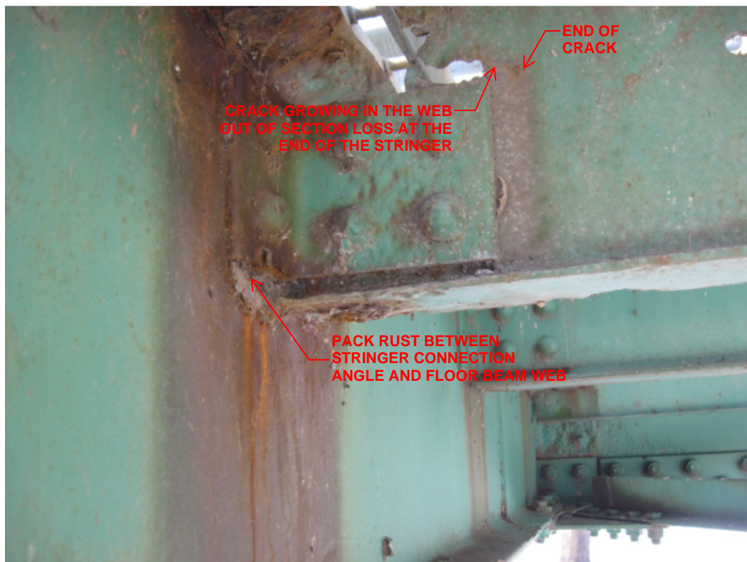
Figure 2: Crack at Stringer End
