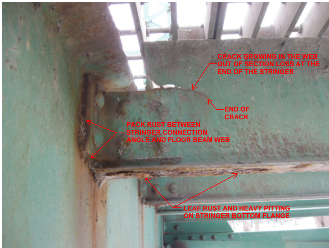
Figure 1: Crack at Stringer End
