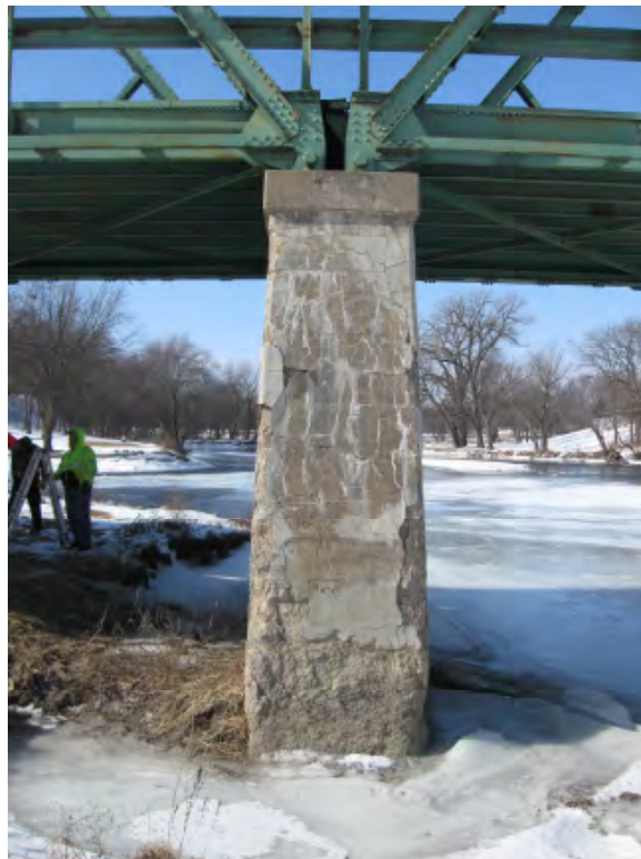
Figure 22 – Deterioration at South Pier
