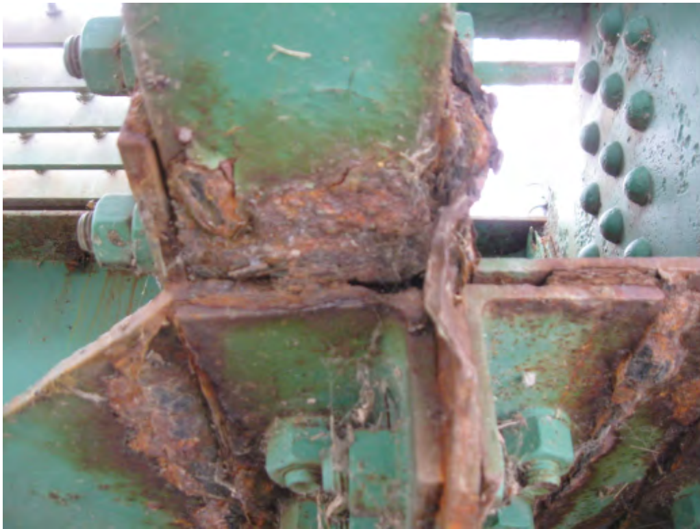
Figure 13 - Example Deterioration at Bottom Chord
