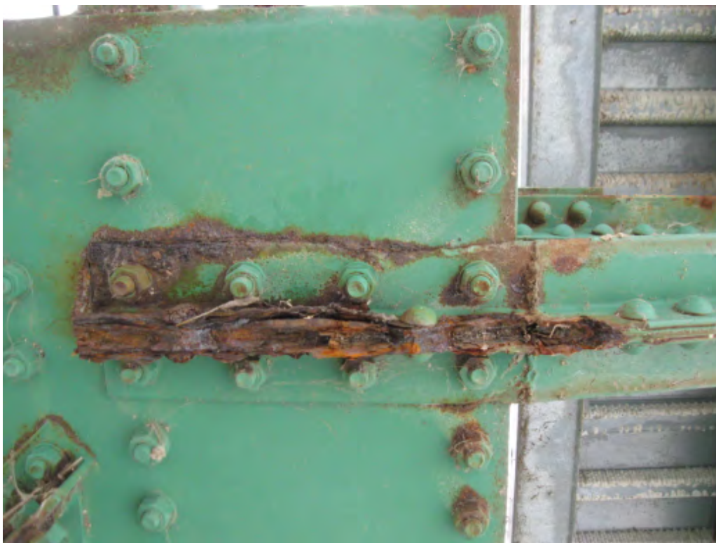
Figure 14 - Example Deterioration at Lower Sidewalk Connection
