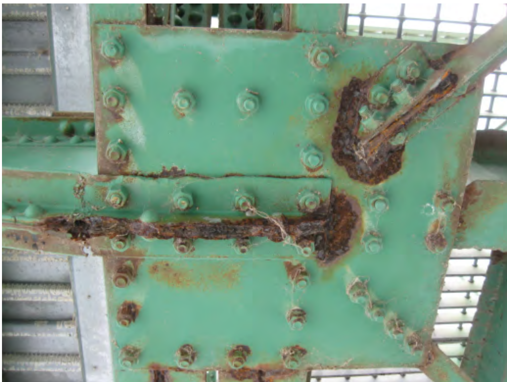
Figure 16 - Example Deterioration at Lower Horizontal Gusset Plate
