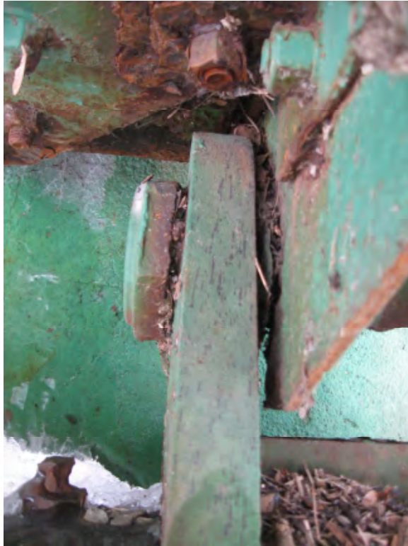
Figure 5 - Example Deterioration at Bearing
