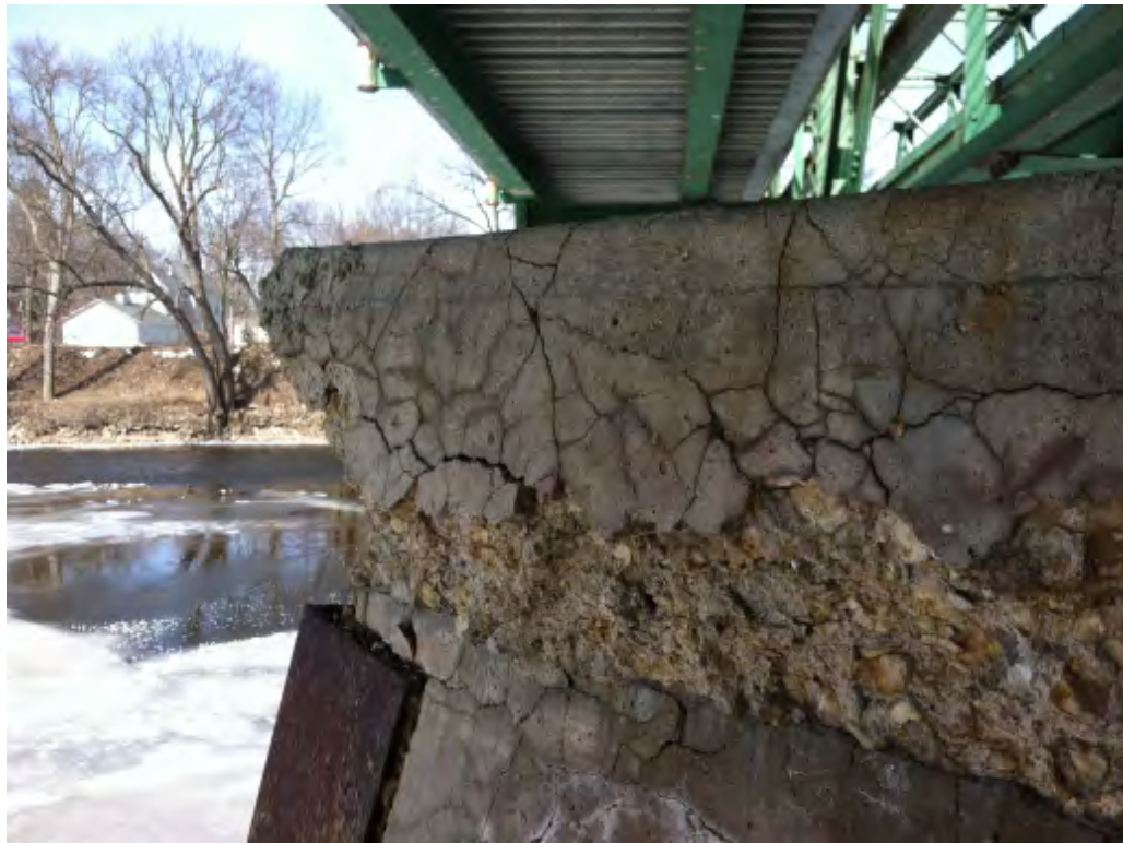
Figure 23 – Deterioration at South Pier (2013 Photo)
