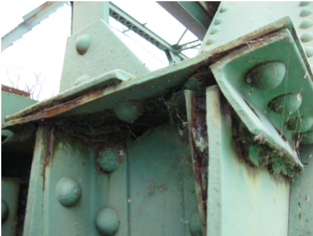
Figure 11 - Example Deterioration Above Bearing
