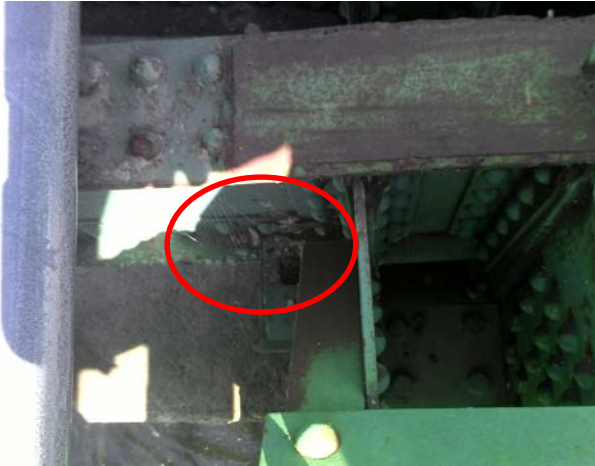
Sidewalk Bracket @ N. Pier – Section loss through bott. Flange
