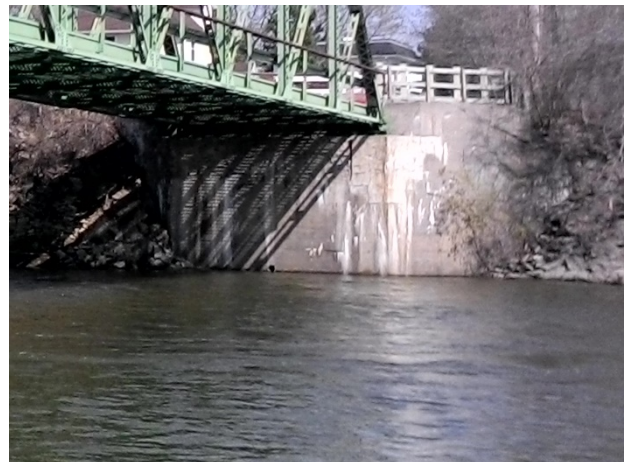
North Abutment – Major cracking w/ efflorescence
