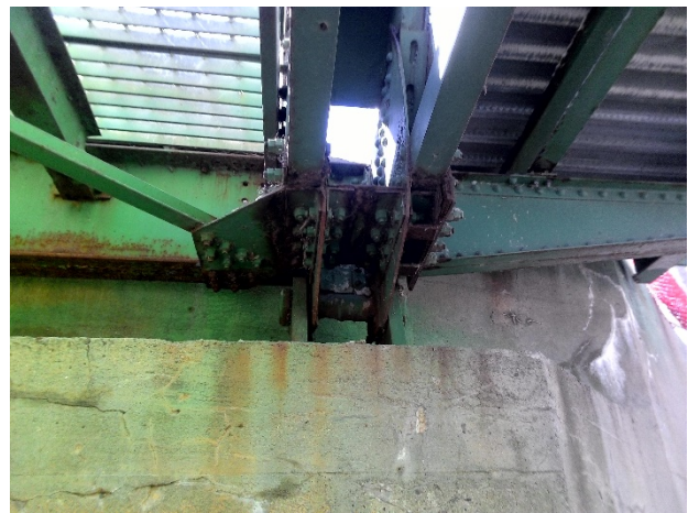
South Abut. Seat – Major cracking w/ efflorescence
