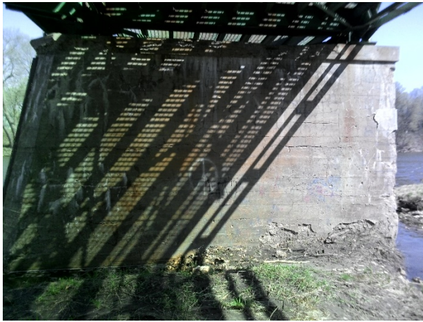
S. Pier, S. Wall – Delamination, spalling, cracking w/leaching
