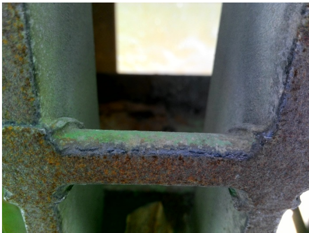
Typical corrosion on deck grating
